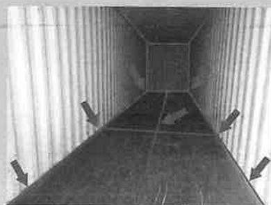
床板・内壁・天井
